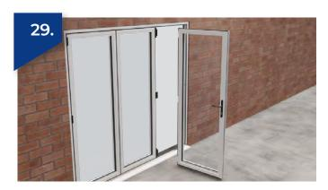
Starting with the single 'traffic' sash if available. Open and remove the screws from the hinges, fully supporting the sash while this is done. Lift carefully and place securely out of the way to prevent damage.
