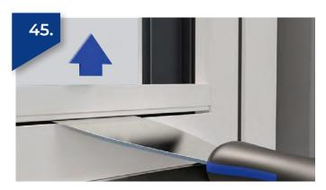
Push down on tool to disengage bead.
